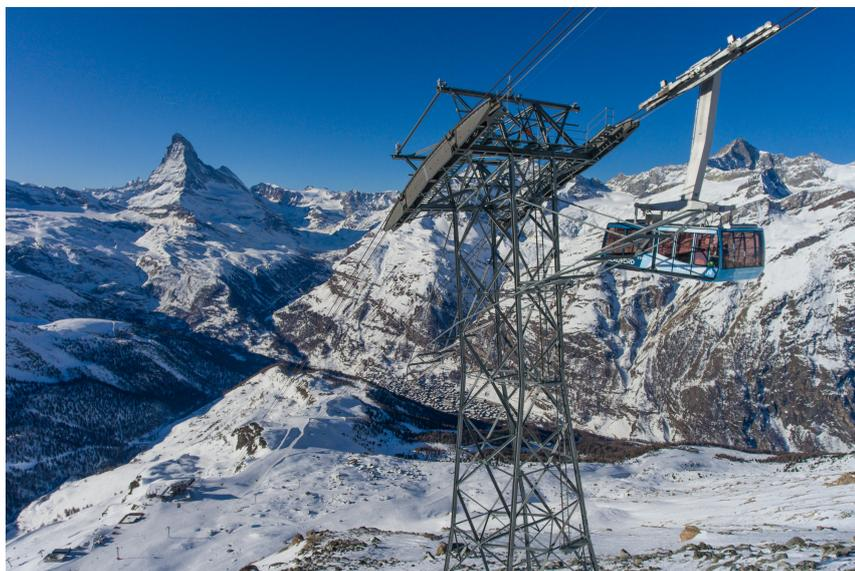
Thawing permafrost due to global warming or other changes in the subsoil can lead to instability in mountain railways and restaurants. Zermatt Bergbahnen decided to monitor this problem with permanent GNSS and laser distance measurements on various mountain railway masts. Depending on the task, the GNSS sensors were attached to the mast foundations or the yoke. The laser distance sensors permanently measure distances between large support feet in order to detect uneven deformations.
