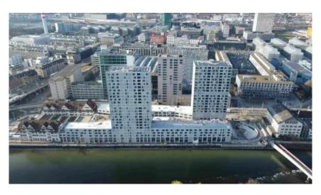
A new building with 220 apartments was planned and constructed in the area of the old tram depot at Escher-Wyss Platz in Zurich. A new, continuous tram depot was built on the ground floor of the two high-rise buildings, which placed additional demands on the structural and stabilization concepts.
