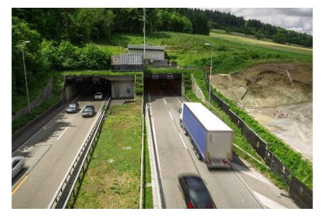
To eliminate a bottleneck on one of the busiest stretches of road in Switzerland, a third tunnel tube was built at Gubrist (length: 3 km) near Zurich.
