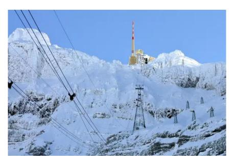
At 2,502 meters above sea level, the Säntis is the highest mountain in the Alpstein (a mountain range in eastern Switzerland). In mid-January 2019, heavy snowfall on the north side of the Säntis caused a massive avalanche. The 54-meter-high support 1 of the **Säntis Schwebebahn**, which runs from Schwägalp at 1,350 meters above sea level to the Säntis excursion summit, was severely damaged. Following this incident, passenger transport had to be suspended.
