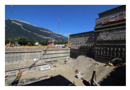
The SUN expansion project at the Cantonal Hospital of Graubünden included a new building with an underground parking garage. The excavation pit, which was up to 22 m deep, was partially adjacent to the existing ward block. In addition, a channel for energy supply was driven under the existing buildings, which house an MRI unit and an operating theater.
